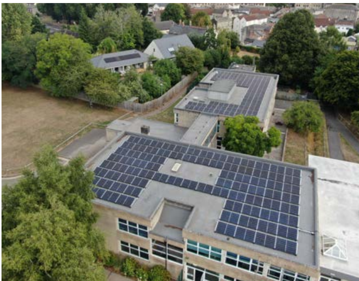
114 kW Solar PV Installation at Somervale School – Installed August 2022
