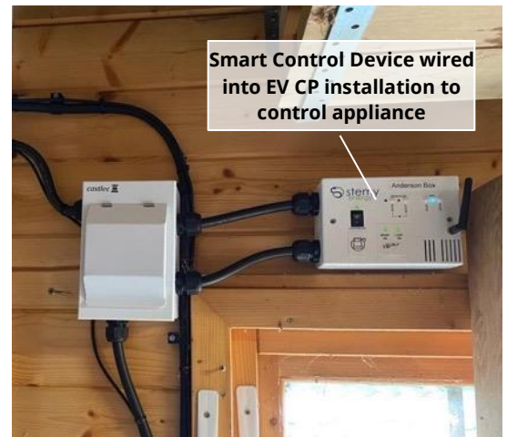
Figure 2: Example EV ChargePoint Installation
